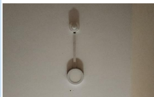
Sensor based lighting in washrooms
